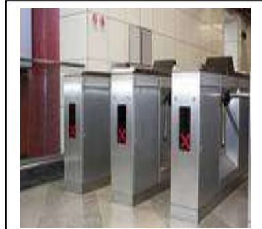
Figure 11: Proximity Card Reader
