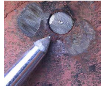
Fig-26 Broken bolt
